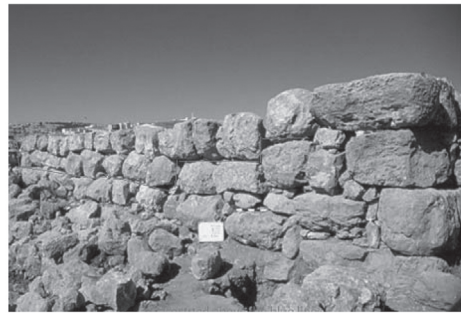
D: Reconstructed the upper part the east wall of structure I
